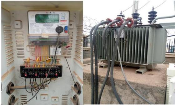
**Figure 1.** CT-operated metering system
