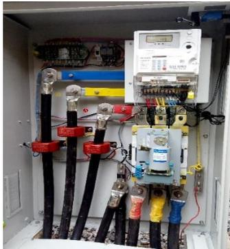
**Figure 4.** Low-voltage CT-operated prepayment energy meter
