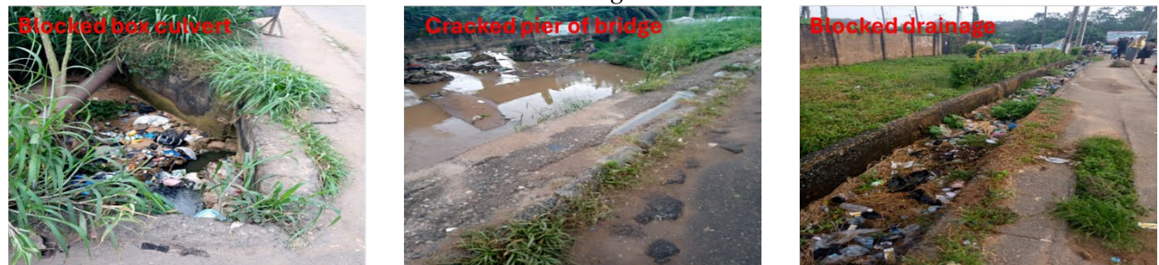
Plate 3: Drainage condition survey
