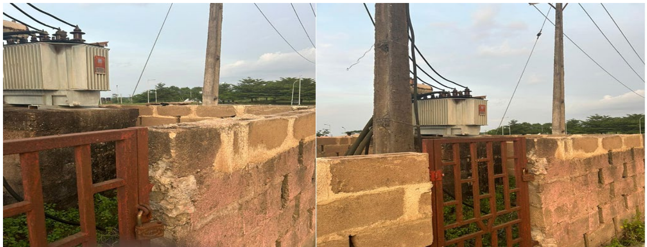
Figure 4. Performance testing of the developed system at a typical substation with the developed intrusion detection system installed
