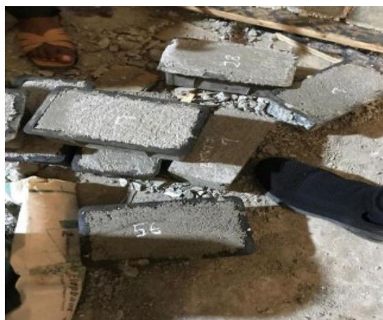
Figure 1: Cast Concrete Paver Blocks in Moulds Prior to Demoulding
