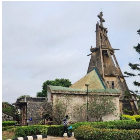
Plate 2: An angular view of the Chapel showing the tower, roof (with incorporated barrel vault) and one of the side entrances.
