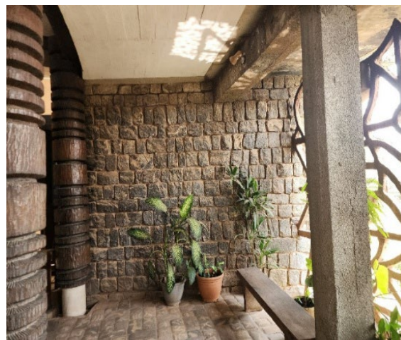
Plate 5: The Side Entrance Foyer indicating extensive openness to maximum ventilation
