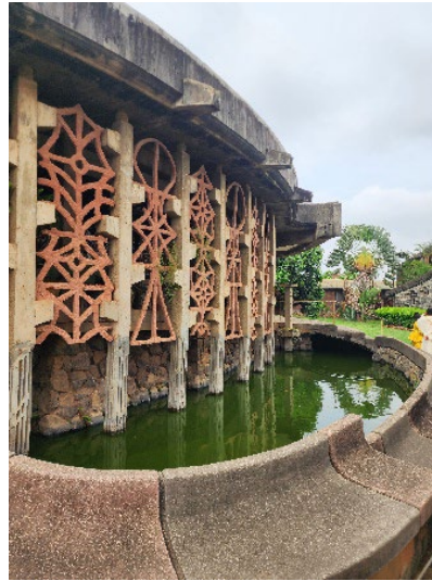
Plate 6: Picture showing the installed moat on one side of the Chapel
