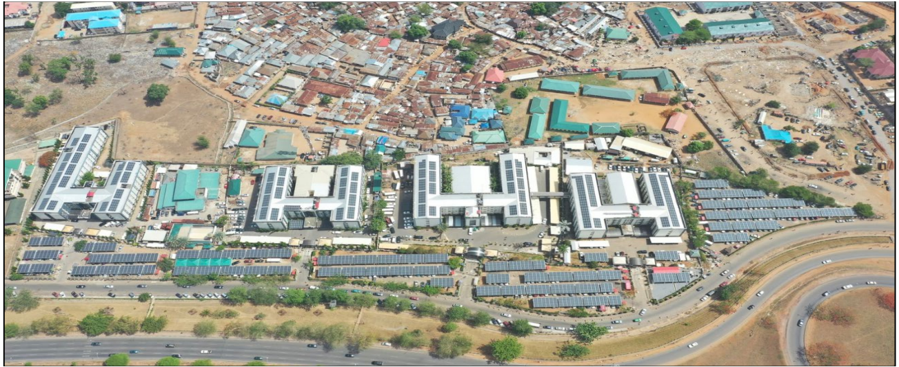
Figure 1: Aerial view of the 1.54 PV / 2.28 MWh storage microgrid in Mabushi, Abuja
