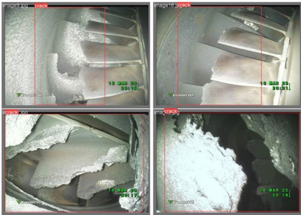
Figure 4: Crack Detection Result
